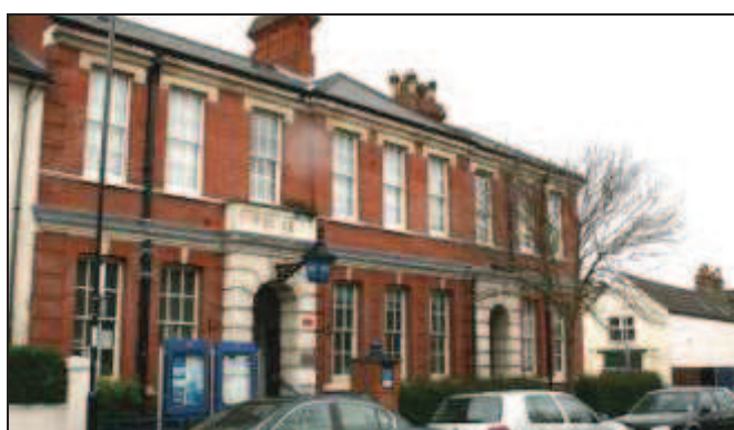
Brockley Police Station
